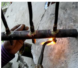
Figure 10. Covering top of the condenser.
