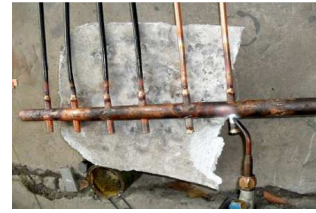
Figure 11. Attaching Copper pipes to the header pipe.
