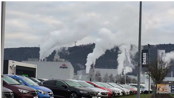
Figure 2. Wet steam emissions from a paper and cardboard factory. 1 m 3 of steam per second contains a thermal energy of 1.56 MW (Image: G. Muller).
