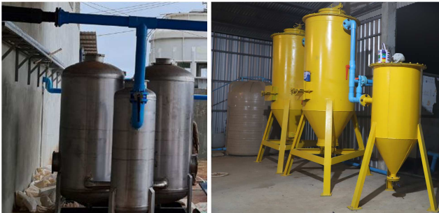
Figure 2. The Chinese desulfurizing system (left) installed on a large-scale pig farm in Preah Sihanoukville Province and the BTIC desulfurizing system (right) installed on a large-scale pig farm in Kampong Thom Province.
