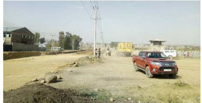
Figure 6. Utilities poorly placed at the center the Mekelle-Samre road to Abune-Aregawi Lachi Church road project 2 years prior to its commencement, Mekelle, Ethiopia, May 31, 2019.
