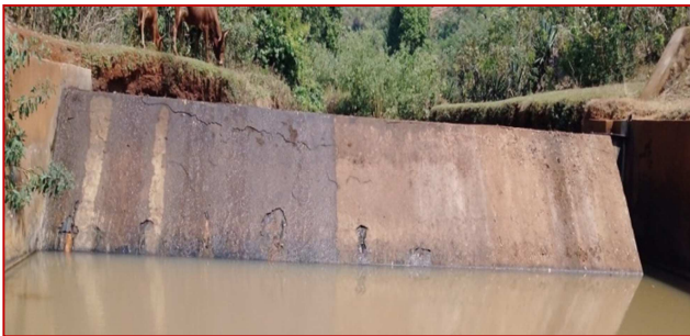
Figure 7. Lack of under sluice gate.
