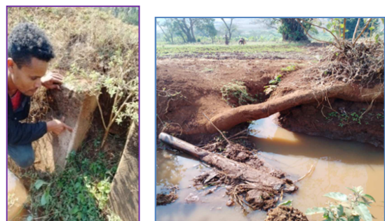
Figure 10. Clogging of turnout structure.
