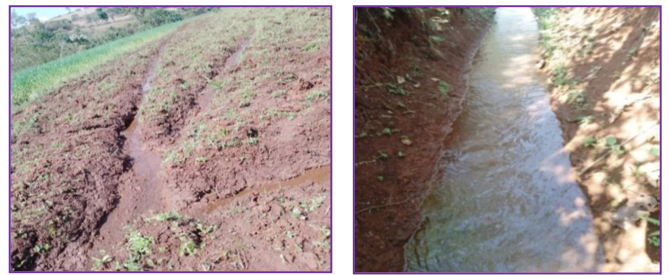
Figure 9. Highly seepage due to the unlined canal.
