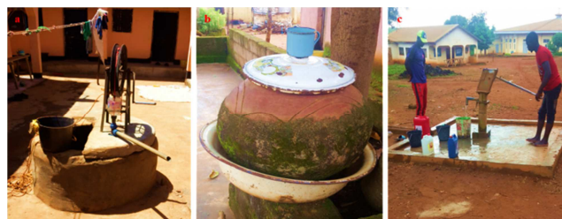
Figure 1. Drinking-water supplies sources unprotected/traditional well (a); clays pots water (b) hand pumps/boreholes (c).
