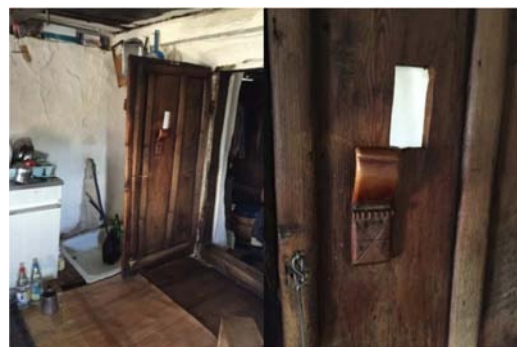
Figure 19. Doors on the room in the Tresnjo family house (Door detail – “saving opening” for transmitting light from the “kuca” to the room).
