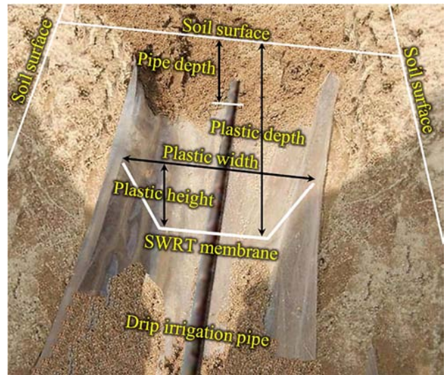
Figure 13. Plastic film and drip irrigation pipes installed under soil surface.
