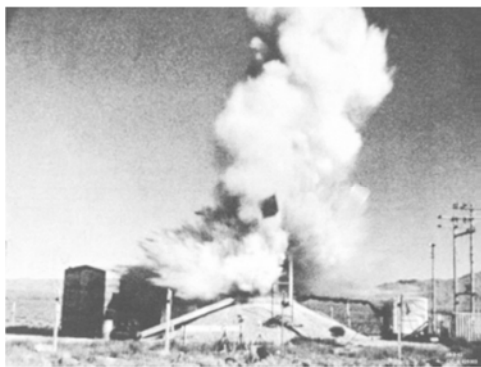
Figure 20. Borax-1 criticality and explosion test in 1955 resulted in a much larger explosion than expected due to previously unknown hydrogen explosion effects (McLaughlin, et al. [49]).
