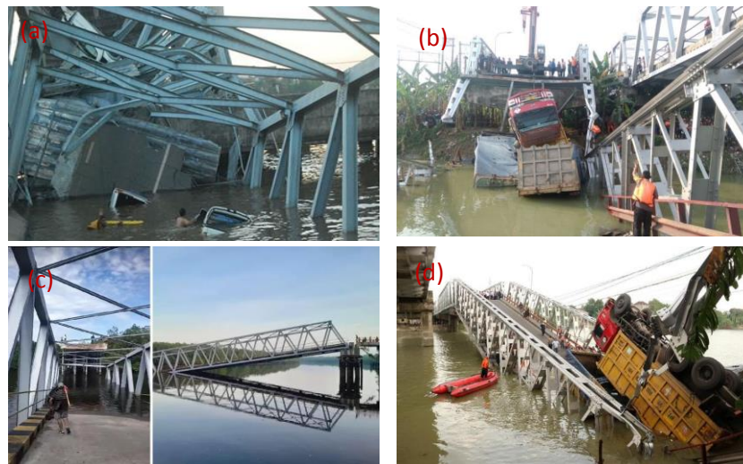
Figure 1. The steel bridge collapsed in Indonesia; (a) Kutai Kartanegara (2011), (b). Babad Widang, Lamongan (2018). (c). Parawang, Riau (2023); Aceh, (d). Pematang Panggang, Palembang (2019).
