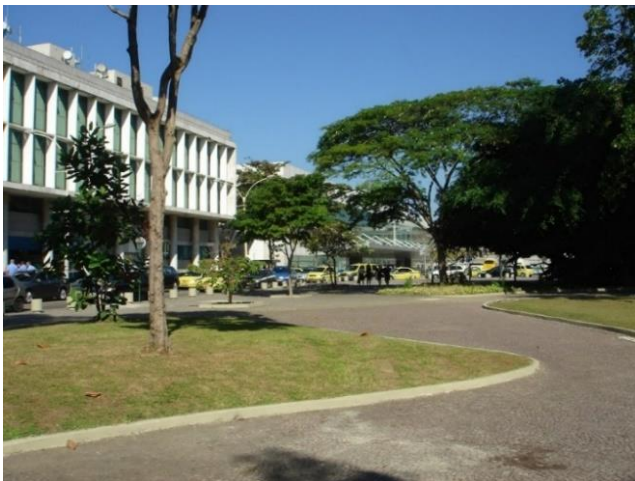
Figure 3. Senator Salgado Filho Square in front of Santos Dumont Airport, RJ. Photo: Alda Ferreira, 2023.
