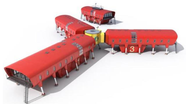
Figure 3. Aerial layout of the modular, elevated living and research wings of the Juan Carlos I, Antarctic Research Station. Designed by Hugh Broughton Architects & ARC. Source: https://spacearchitect.org/portfolio-item/juan-carlos-1-antarctic-base/ . [27].
