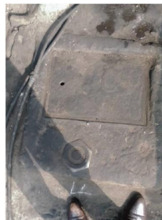
Figure 8. Cement-sealed hydrant.
