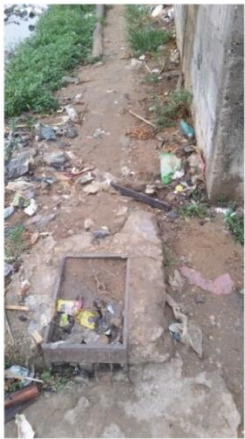
Figure 2. Fire hydrant blocked by mudslides and debris from a gully.
