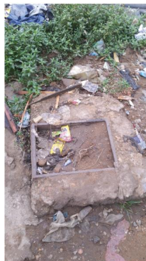
Figure 7. Fire hydrant blocked by undergrowth and sand.
