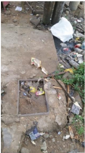
Figure 3. Fire hydrant blocked by mudslides and debris from a gully.
