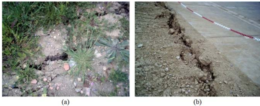
Figure 10. Fissures observed in the soil and near to the road N: 01.
